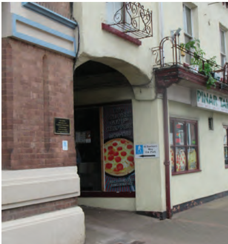
↑ Poor signage to route to car park
