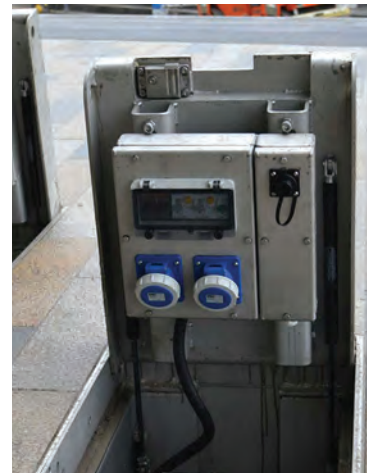
↑ In-ground power supply
