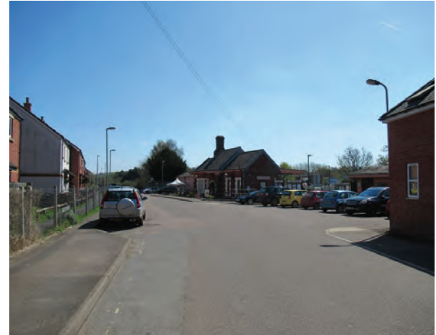
↑ Existing station approach provides an underwhelming gateway
